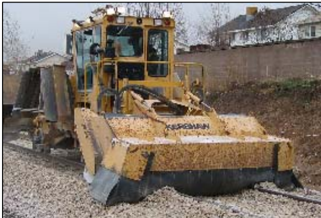
Rail Sweeper and Salvage
