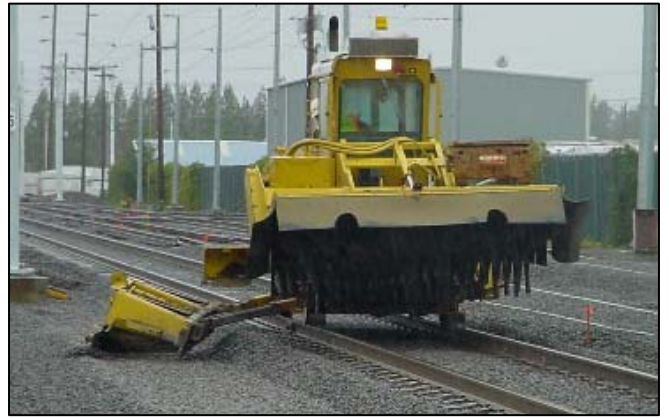
Rail Sweeper and Grader
