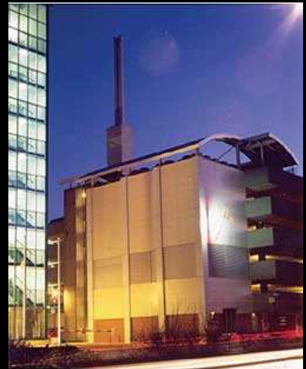
Woking town centre demonstrating combined heat and power
