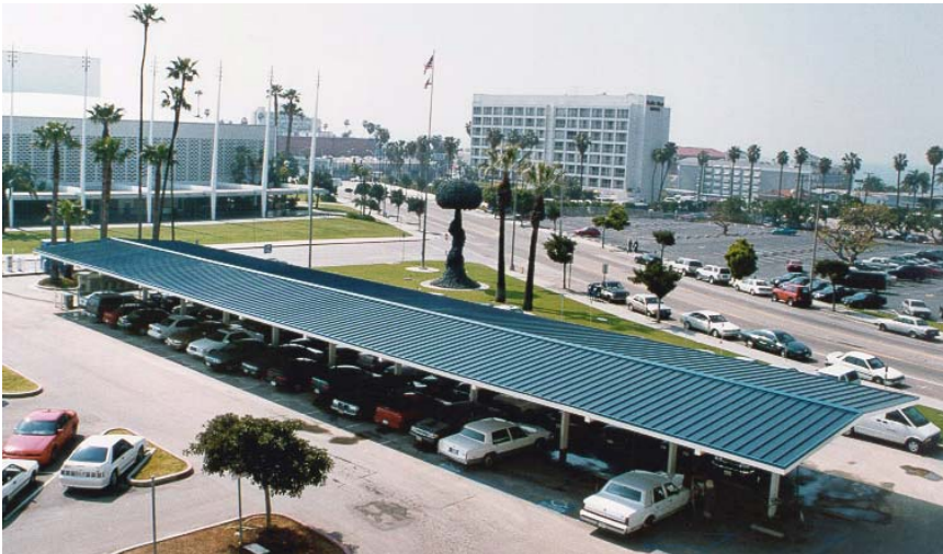
30 kW EV Charging Shade Structure
