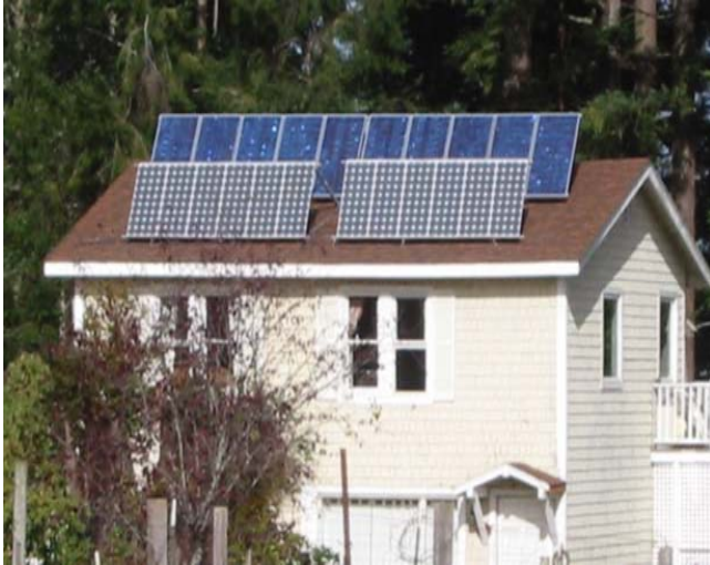
Modules installed on racks
