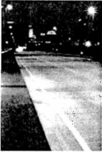
Concrete pavement reflects up to 27% of light. Black asphalt pavement reflects only 5% of light.
