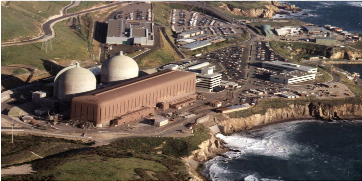
Diablo Canyon nuclear power plant
