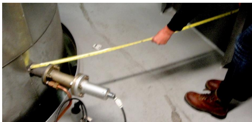
Figure 2-3 Platform space available for equipment (smoke meter shown)
