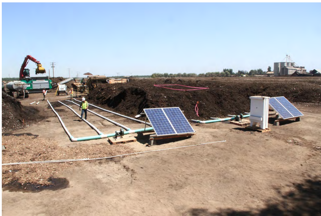
Photo 6: View of project with completed eASP zone 1 on right, and aeration pipes in place for Zone 2. Zone 1 photovoltaic system is complete; panels are in place for Zone 2.
