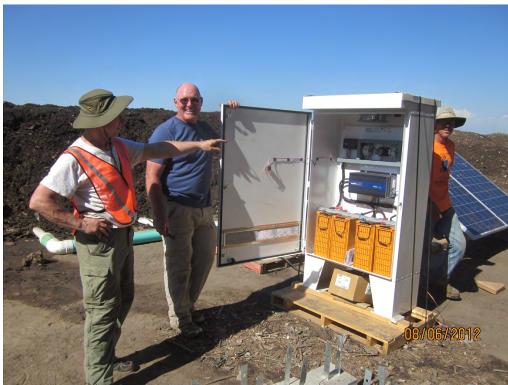
Photo 8: Interior of the power array box. From bottom to top: batteries, inverter, timer and switches, and exhaust fan at very top. From left to right: Harold Ruppert and Peter Moon of 02 Compost, and Kevin Barnes, City of Bakersfield.
