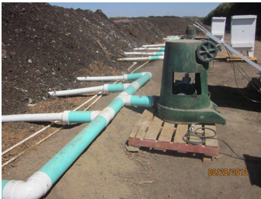
Photo 5: Completed aeration manifold showing 6" pipes, connectors and step down to 4" pipes. The blower is protected inside the modified trash container.
