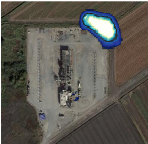
Figure 2: LeakSurveyor false color image of a leak from a gas storage facility; blue represents a methane plume.
