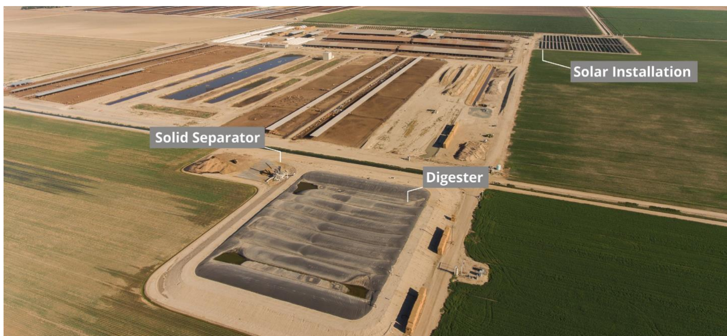
Figure 10. California climate-smart dairy with a digester, manure solid separator, and solar installation.
