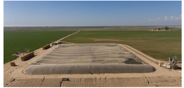
Figure 11. Digester on California dairy farm.
