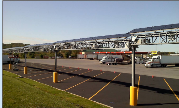
Fig.2: 20 kW Solar Array Pilot #412 - White Pine TN
