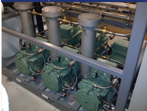
PHOTO 2 Transcritical CO 2 compressors and oil separators.
