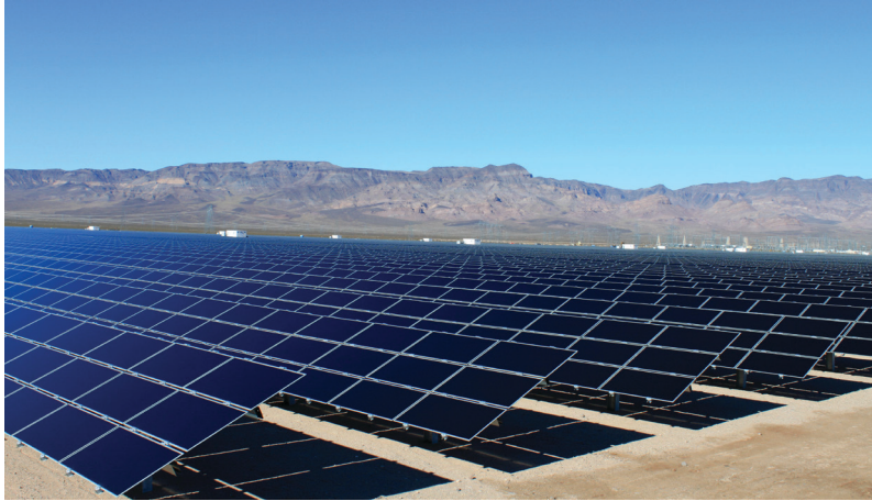
Solar Electric Power Generation
