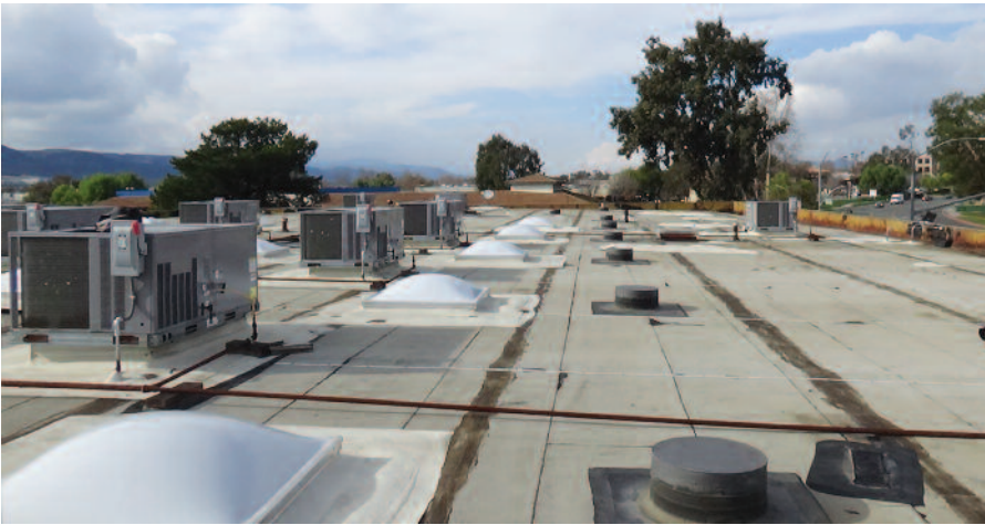
The single-ply membrane on the original BUR roof had been patched many times but was deteriorating and leaking.
