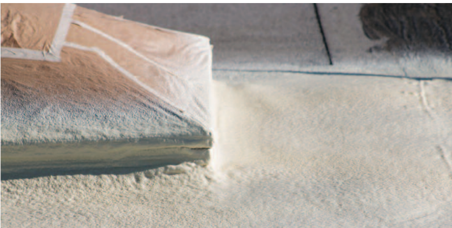
CcSPF's unique ability to contour and seal around skylights and the many other rooftop protrusions made it an ideal solution.
