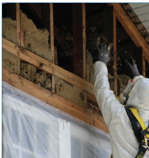
Removing existing cellulose insulation that can slip down the stud cavity, reducing effectiveness over time
