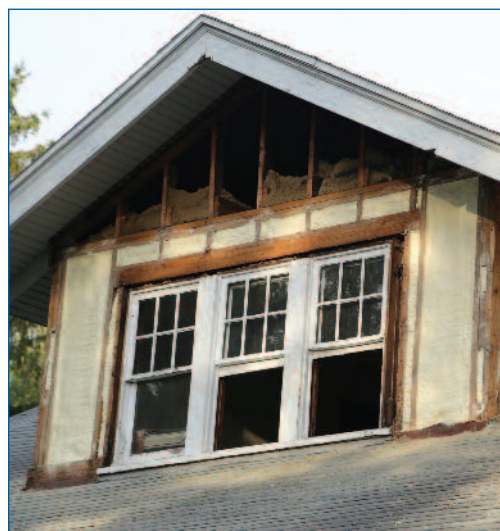
After spray foam insulation installation
