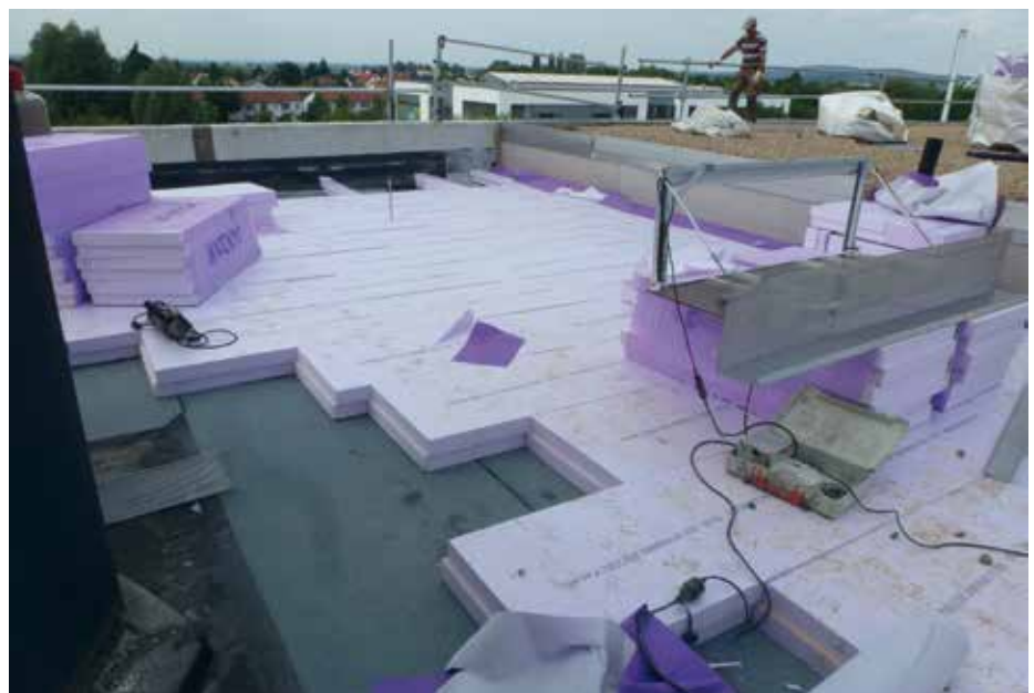
Inverted roof insulation with JACKODUR Plus for University of Applied Sciences in Lemgo
