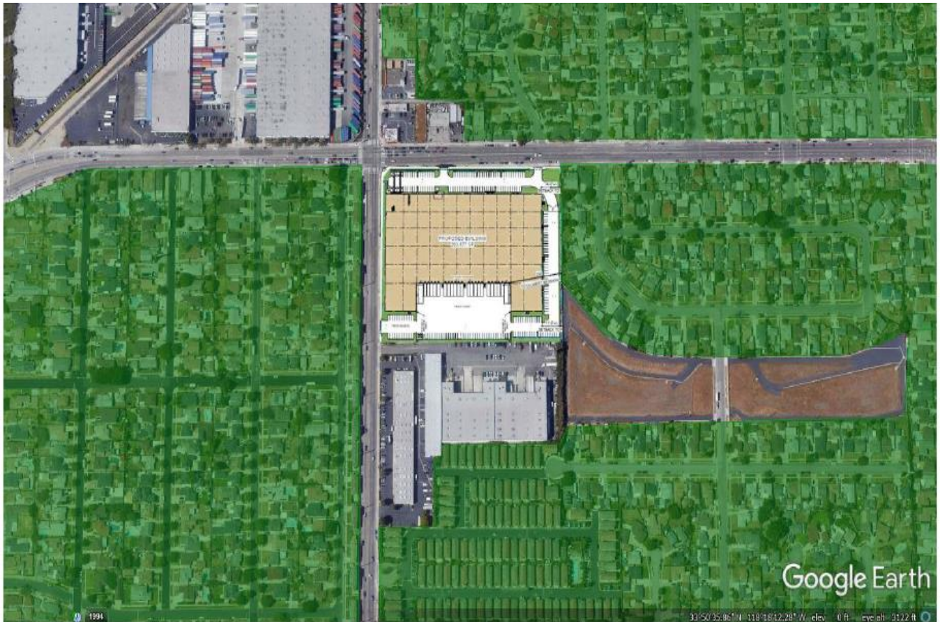
Image of the proposed Project and adjacent land uses, with residential uses highlighted in green.
