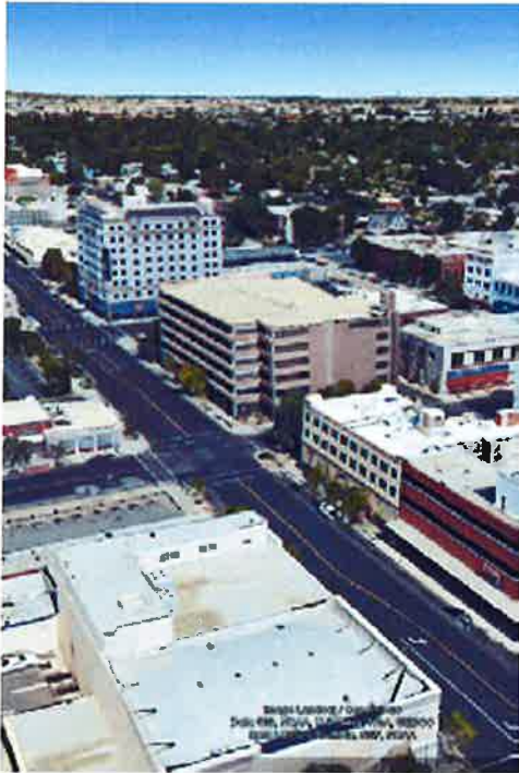
Bakersfield Downtown Parking Garage
