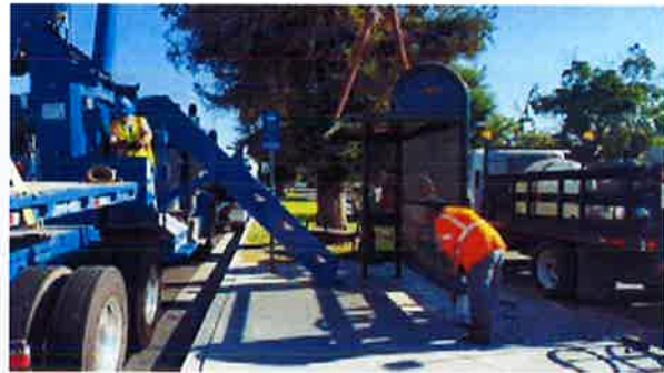
Installation of new bus stop
