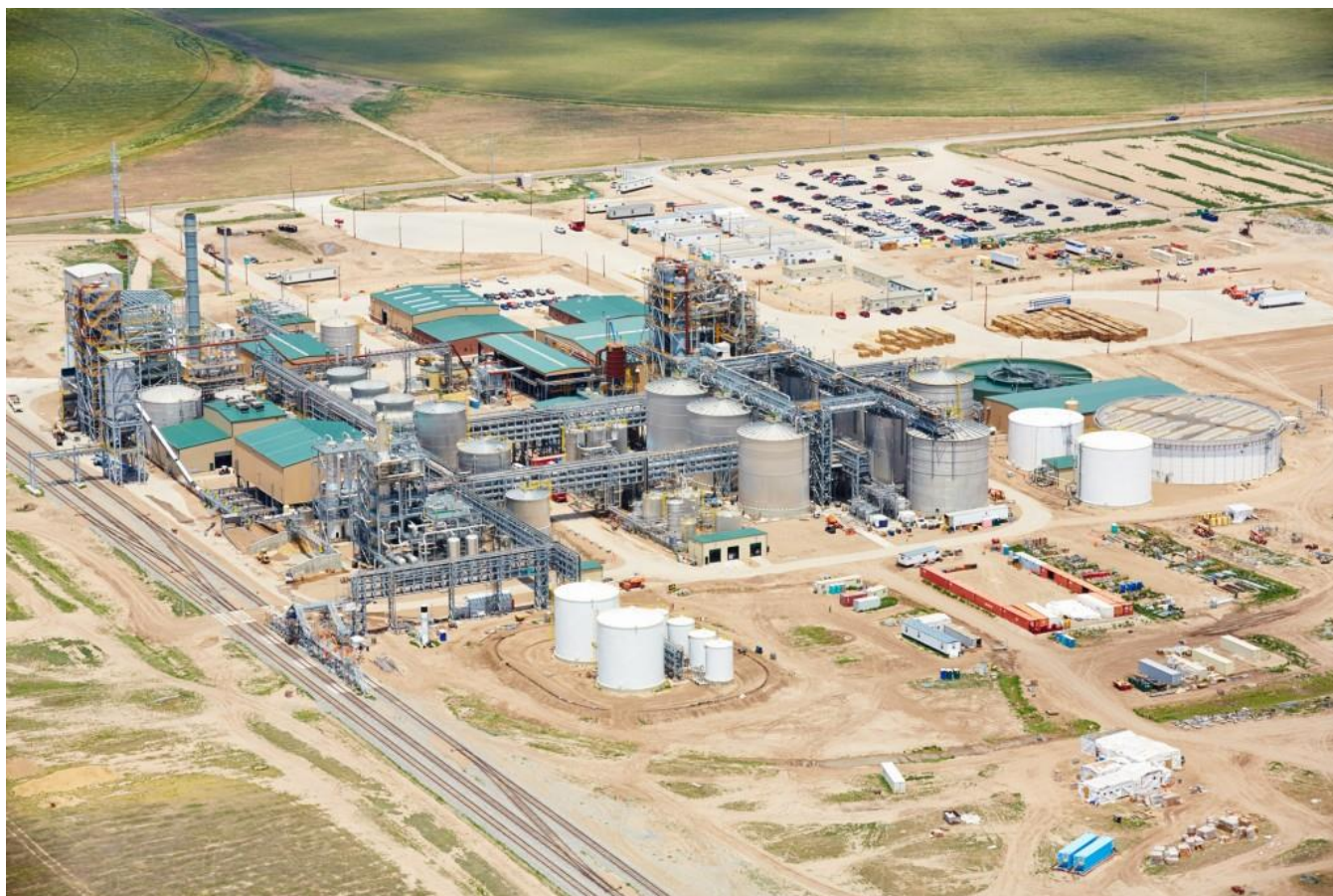
Abengoa's plant in Hugoton Kansas will produce 25 million gallons of cellulosic biofuels and 21 MW of electricity per year – enough to power the plant and sell some back to the local Stevens County community. Photo credit: Abengoa
