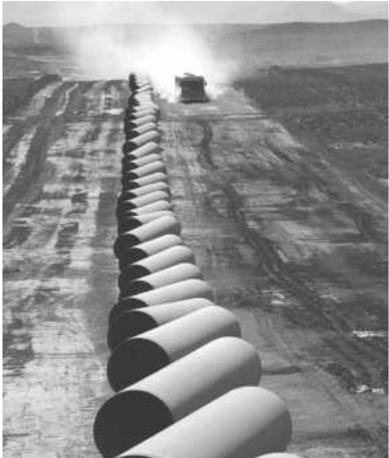
Segments of the Baku-Ceyhan pipeline await assembly.
