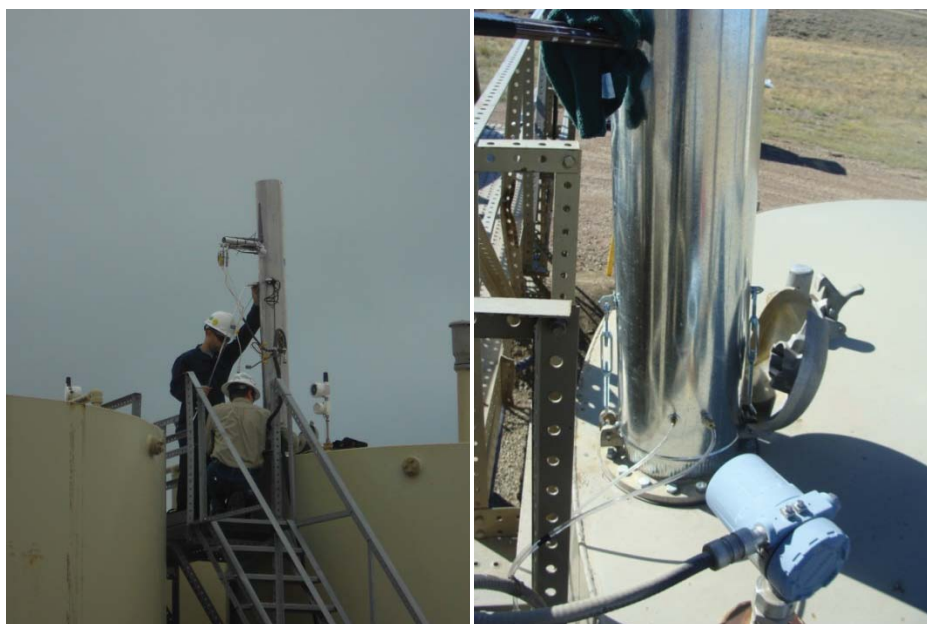
Figure S3-1. Temporary Stack on Blowdown Site Tank Hatches
