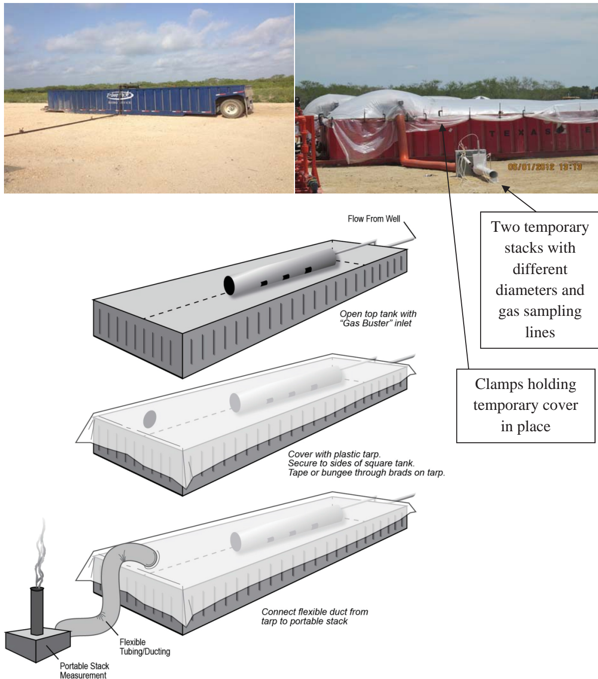
Figure S1-2. Open top tank used in Step 1 of flowback using the equipment configuration shown in Figure S1-1. Upper Left: line leading from well to tank; upper right: temporary plastic cover installed and clamped to edge of tank, with exhaust stacks on ground adjacent to tank; lower: Conceptual diagram of sampling system.
