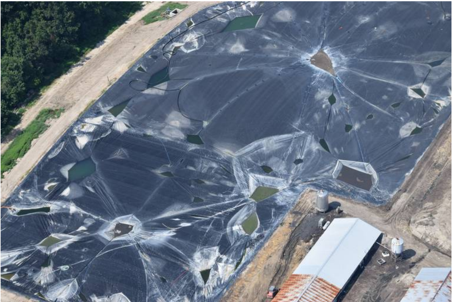
The covering on a Wayne County lagoon broke open in late May, sending more than four swimming pools' of foam across White Oak Farms in Fremont. The damaged anaerobic digester is shown here on August 3. Samantha Krop Sound Rivers
