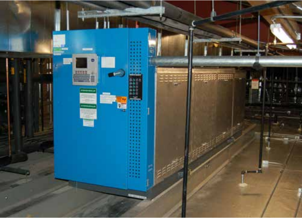
In April 2011, Sprouts installed this Hill-PHOENIX Second Nature CO 2 Cascade System
