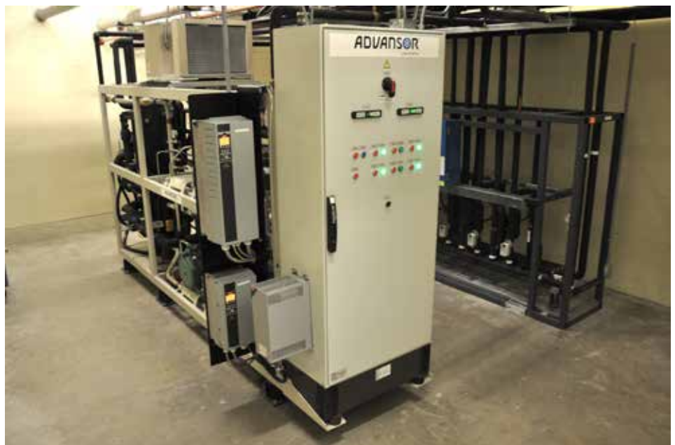
Hill-PHOENIX ADVANSOR Transcritical refrigeration system
