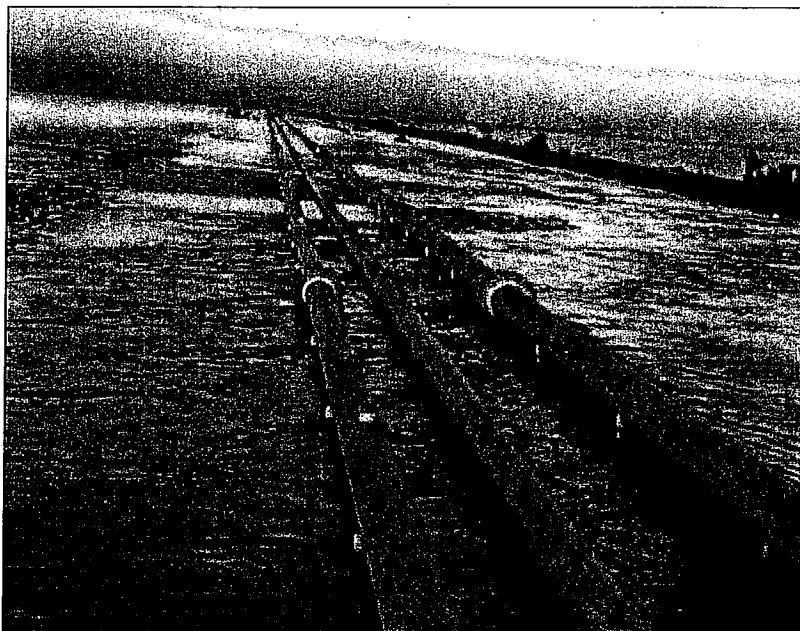
Rising sea levels threaten levees in the Sacramento/San Joaquin River Delta, home to East Bay Municipal Utility District's three primary aqueducts and much of California's water supply. A singular levee breach in 2004, shown here, submerged the district's aqueducts for more than four months.
