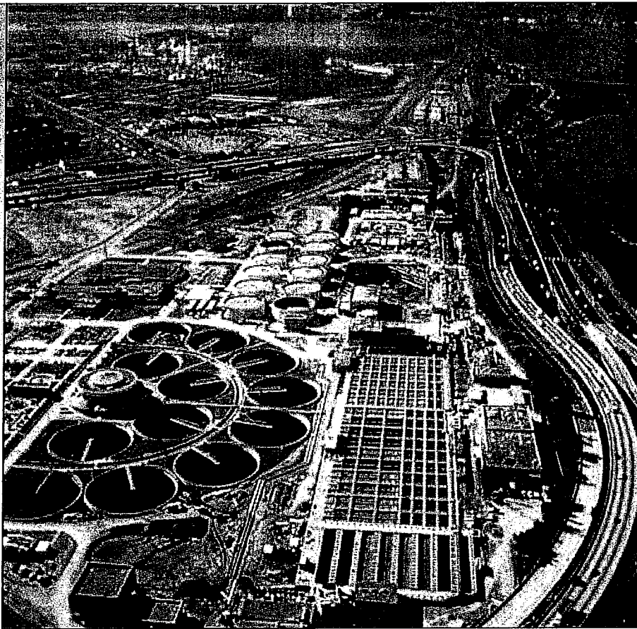
East Bay Municipal Utility District uses available capacity at its wastewater treatment plant to convert trucked-in nonhazardous waste (such as food processing waste and wastewater sludge) to methane, which is used to generate renewable energy.
