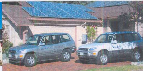
110kWh/day PV, 52 kWh of EV batteries
