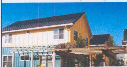
6kW BIPV provides power for Co-Housing and shared EV
