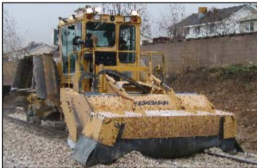
Rail Sweeper and Salvage
