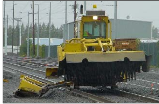
Rail Sweeper and Grader
