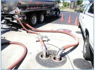
Fuel Transfer From Cargo Tank to UST Volume Meter Installed on Vapor Return
