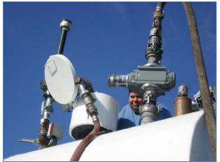
Volume Meter Installed on Vapor Return and Vent Line
