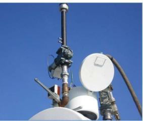
Volume Meter Installed on Vent Line
