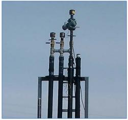
Volumetic Meter Installed on Vent Line
