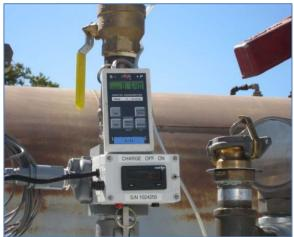
Volume Meter Installed on Vent Line
