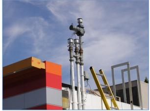
Volume Meter Installed on Vent Line
