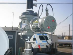
Volume Meter Installed on Vent Line
