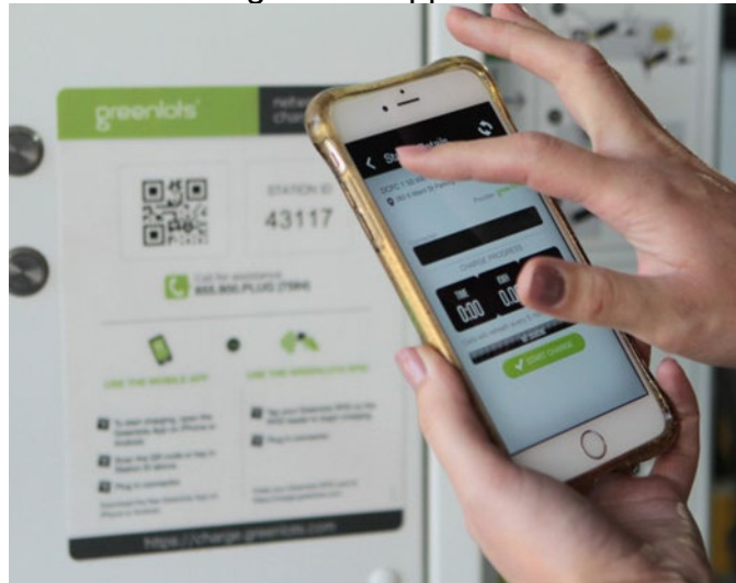
Figure 4 - Sample EVSE allowing mobile application to initiate a charging session
