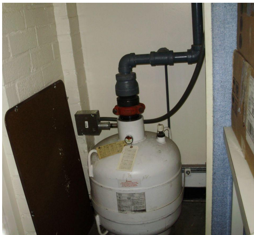
Figure 3-1. Typical Halon 1301 Total Flooding System
