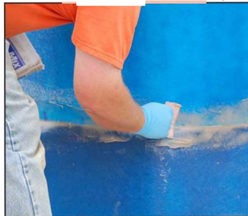
Figure 8: Applying Putty and Catalyst
