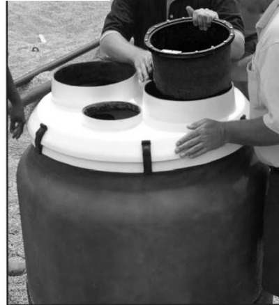
Figure 7: Aligning Multi-Port Sump Shield
