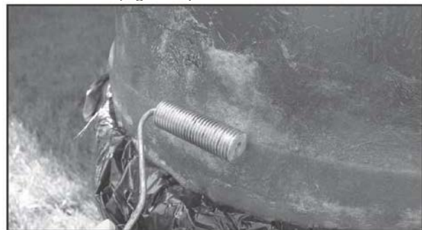
Figure 10: Remove Air Bubbles on Containment Sump
