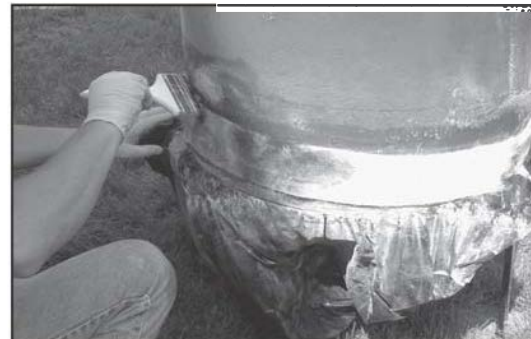
Figure 9: Apply Resin
