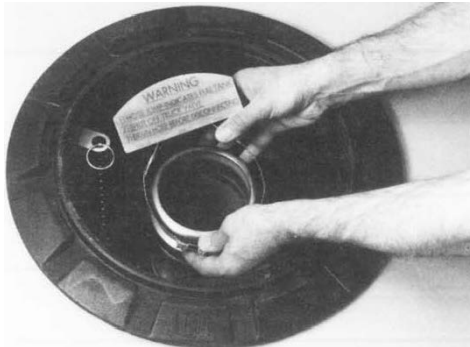
Figure 12: Install Warning Plate
